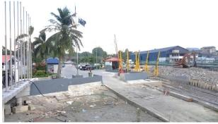
The Club has constructed raised concrete embankments around the renovated slipway to add better protection against potential flooding during periods of exceptional seasonal high tides. A floodgate at the top of the slipway will be mobilised to prevent high tides from overflowing through the slipway onto the carpark areas.
